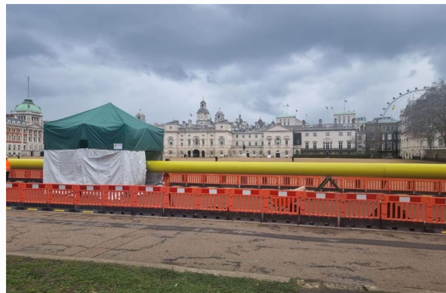
Figure 5.8: 630mm PE insertion on Horse Guards Parade
